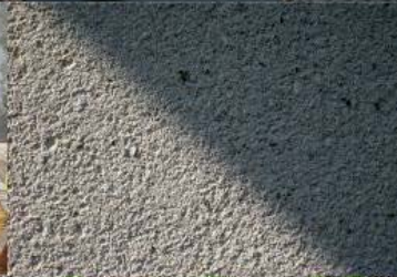
Texture of External Wall
