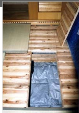
■ Tatami, Cedar Flooring and Recycled Charcoal for Humidity Control
